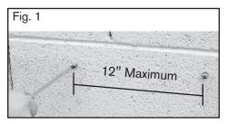
9. Install the bottom two screws and tighten all screws.
