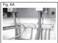
Fig. 6A – Wiring connections to be made inside time clock or electrical panel.
