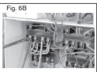
Fig. 6B – Wiring connections to be made inside time clock or electrical panel.
